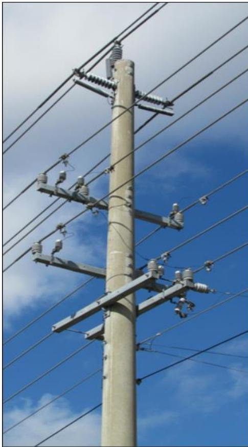
**Figure 7:** Compact 69kV line with double distribution circuit underbuild. Every phase of every circuit is arrester protected. (Lakeland, Florida)
