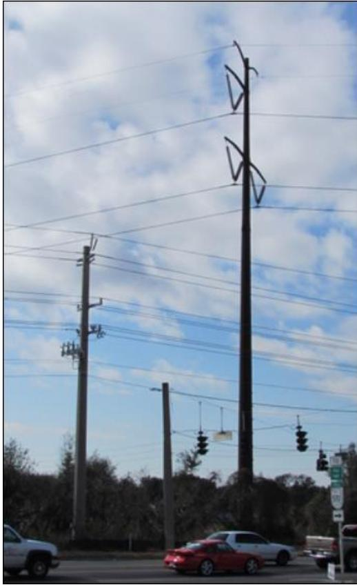
**Figure 6:** This is an example of clearance requirements costing extra for the taller tower. If arresters were used in this case, the tower height could be reduced.
