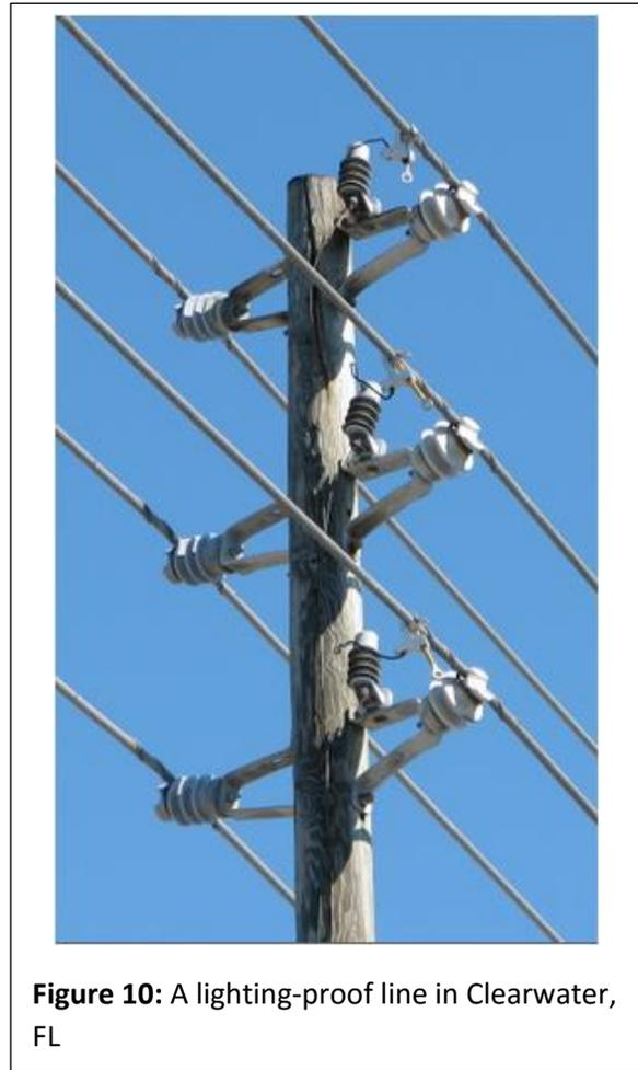
**Figure 10:** A lightning-proof line in Clearwater, FL
